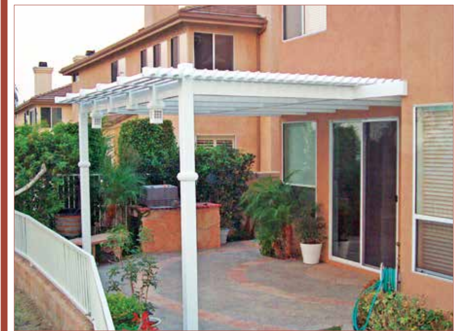
This patio cover is attached to the structure of the house
